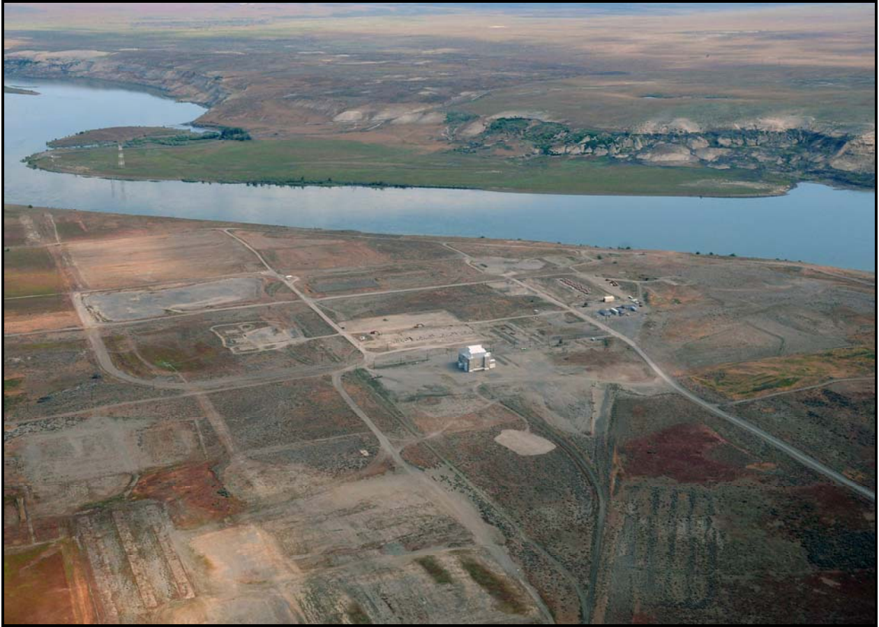
Washington Closure Hanford is remediating 19 waste sites in 100-F Area, home to the third of Hanford's nine plutonium production reactors. (Photo 10)
