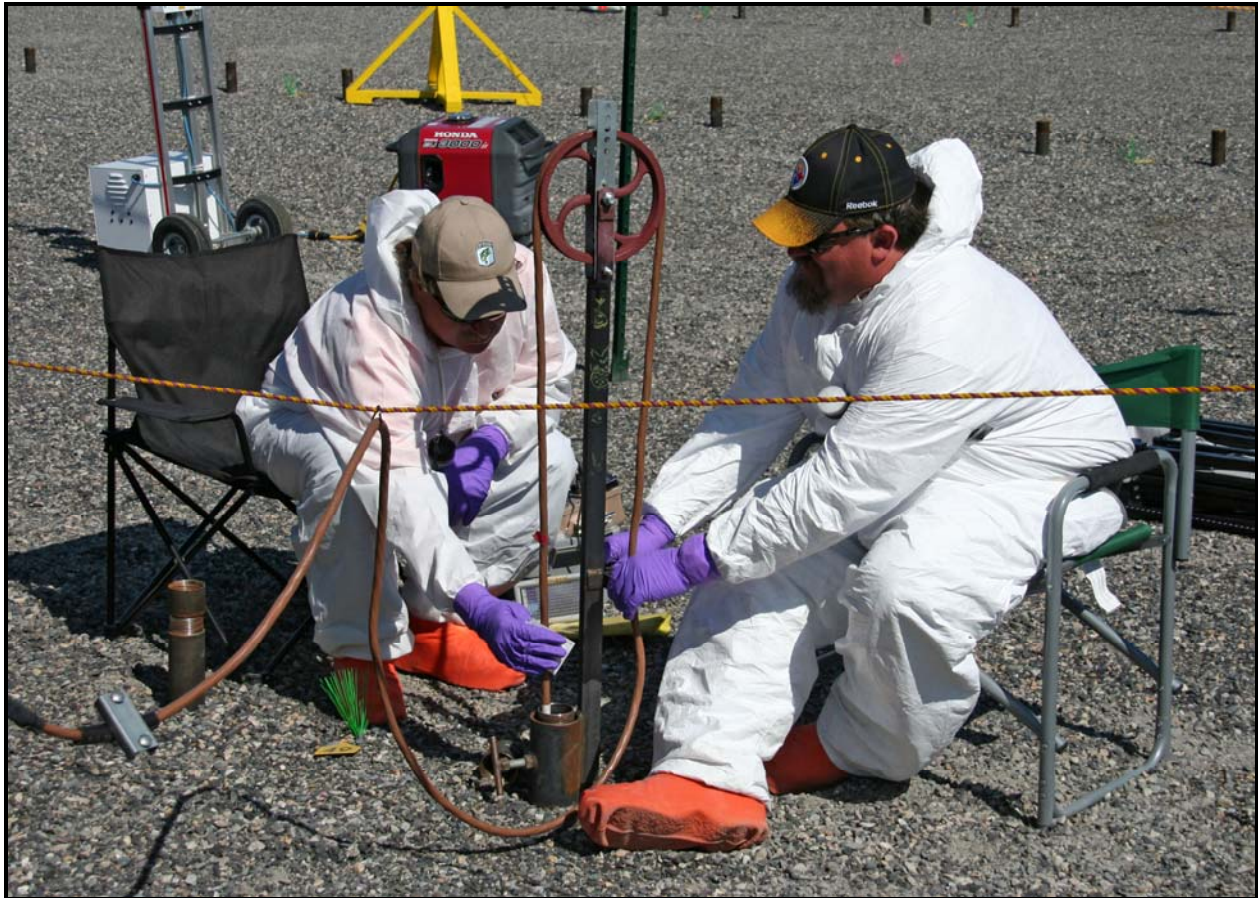
Employees with Washington Closure Hanford subcontractor North Wind Inc. retrieve a multi-detector probe during nonintrusive characterization of the 618-11 Burial Ground. (Photo 10)
