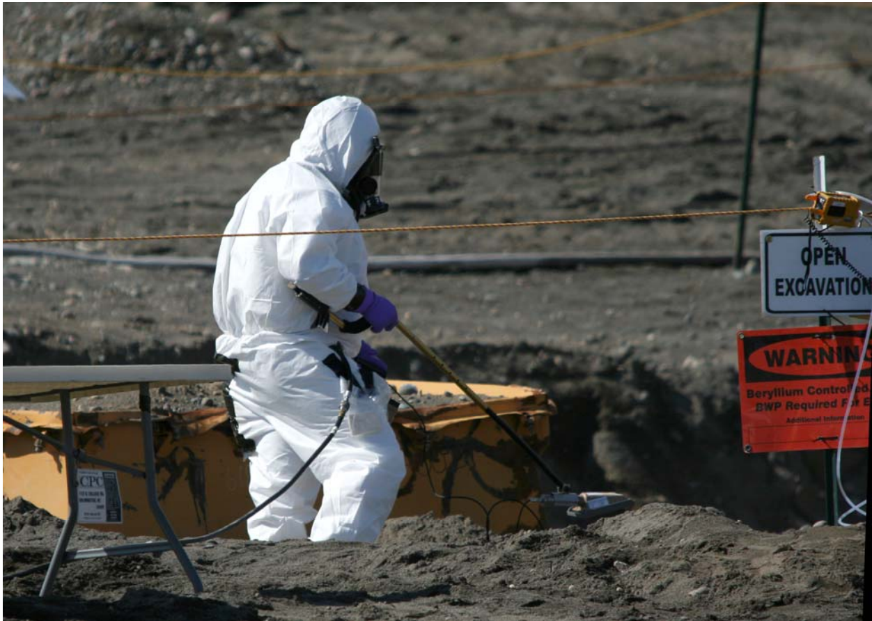
A radiological control technician takes a reading during trench excavation at the 618-10 Burial Ground. (Photo 8)
