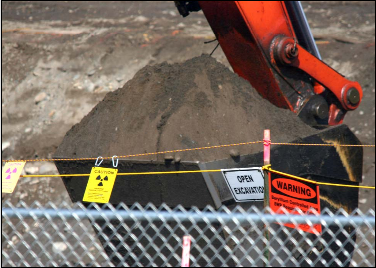
More than 35,000 bank cubic meters have been removed since excavation of the waste trenches began in April. (Photo 6)
