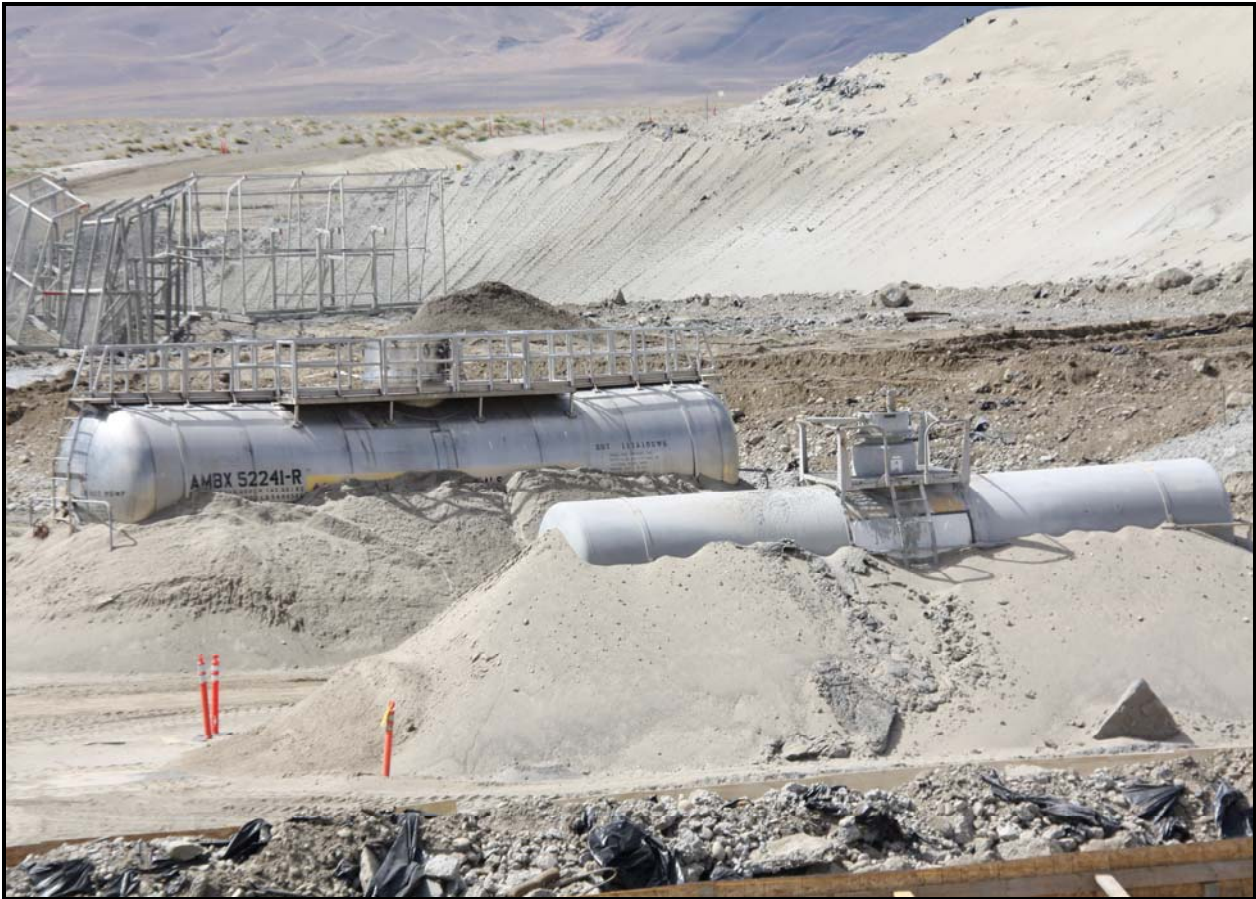
Two Hanford Site tanks cars are being disposed at the Environmental Restoration Disposal Facility. (Photo 3)
