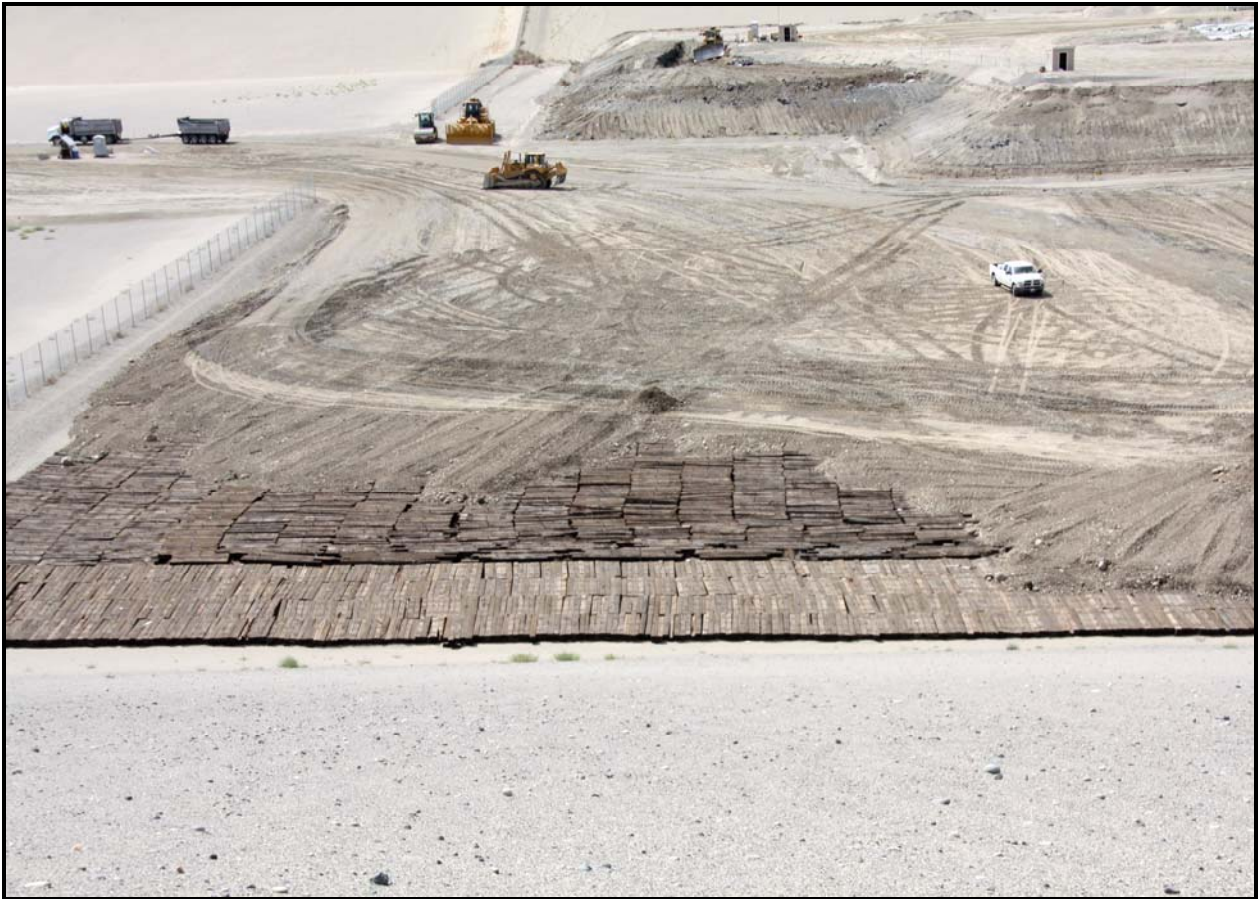
The ERDF disposal team covers nearly 58,500 Hanford Site railroad ties in super cell 9 at the Environmental Restoration Disposal Facility. (Photo 4)
