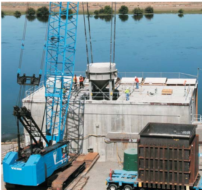
A 96,000 pound box was custom engineered for safe transport of contaminated filter tanks to the Environmental Restoration Disposal Facility.
