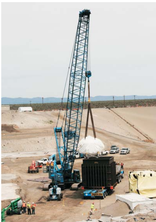
The sand filters from N Reactor will be buried in central Hanford. The T-1 tank will be buried inside the box due to high radiation levels.
