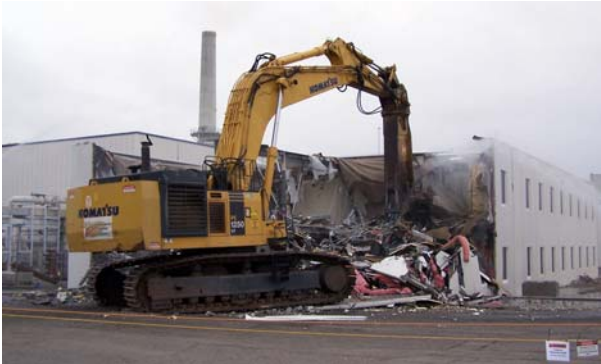
The 324 office wing demolition was completed in 2009.
