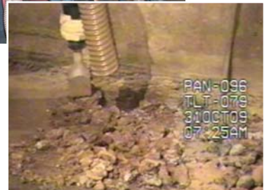
Custom designed tools are remotely operated and used to remove 12,000 curies of radiation from B-cell.
