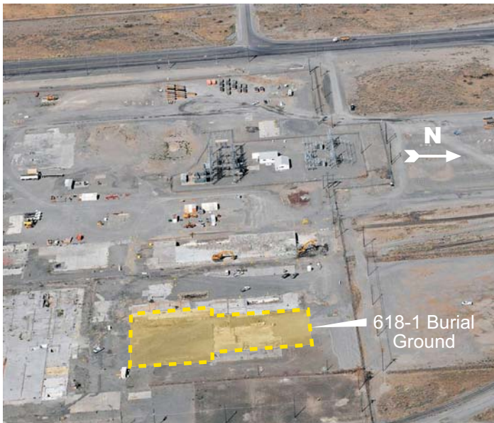
Removal of buildings in the 300 Area provides access to hazardous materials buried a few hundred yards from the Columbia River.
