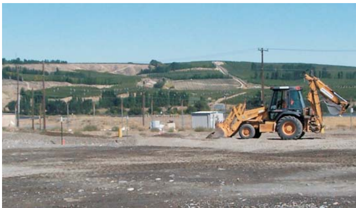
Workers prepare staging areas where contaminated debris will be shipped for disposal. The eastern bank of the river is in the background.
