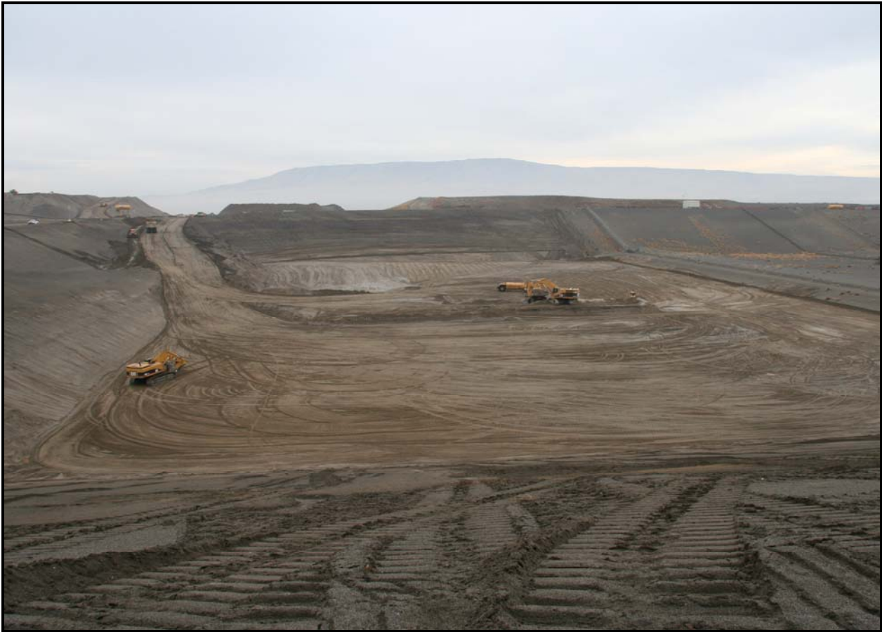
DelHur Industries personnel began excavating the south ramp, upper left, at the Environmental Restoration Disposal Facility.
