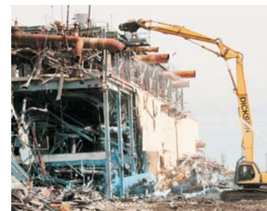
Heat exchanger building demolition March 2009
