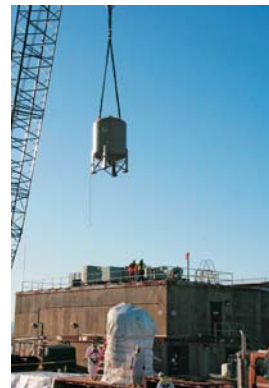
Recirculation building demolition December 2008
