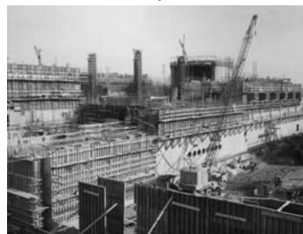
Construction of reactor and heat exchanger building January 1965
