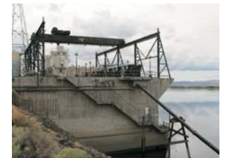
River water pumphouse demolition 2010
