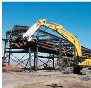
Steam pipe trestle demolition February 2006
