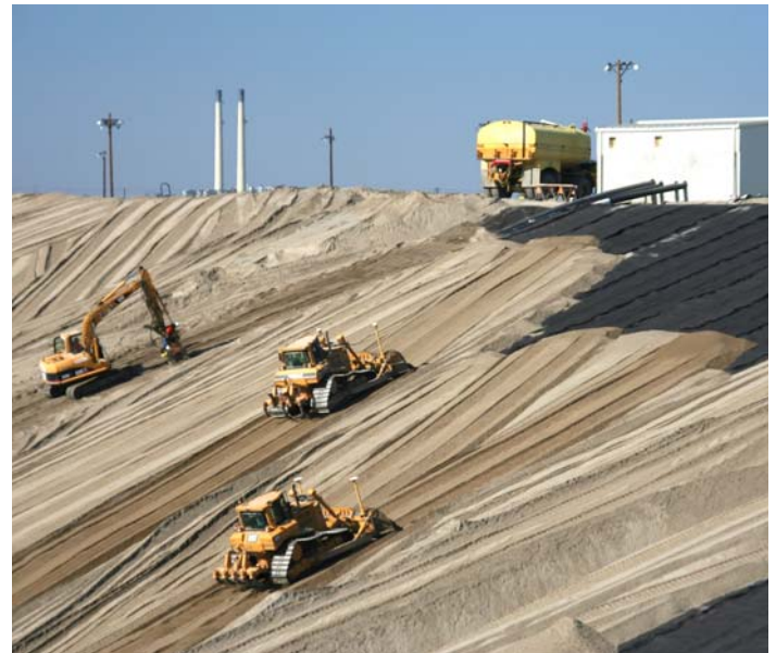
Workers install the operations layer on the north slope of super cell 10.
