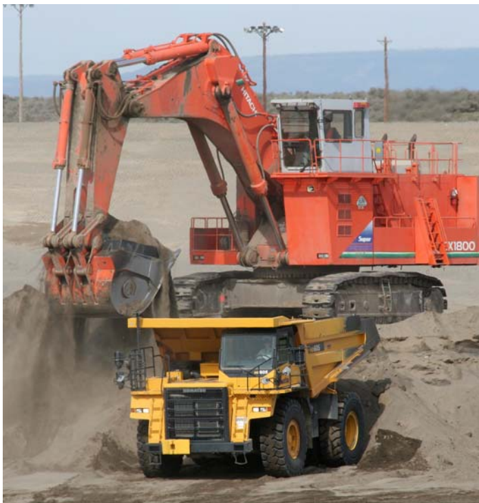
About 1.7 million tons of soil was excavated from super cell 10.
