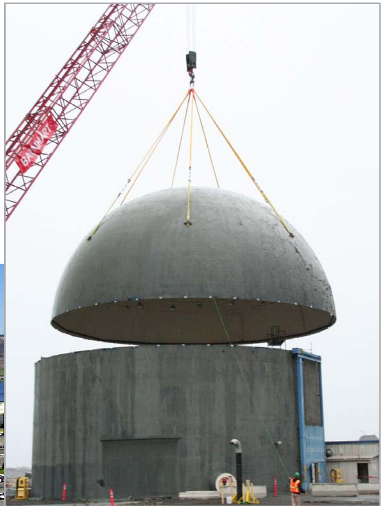
The 67-ton steel dome was removed January 15, 2011.
