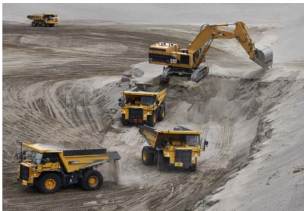
Excavation of super cell 10
