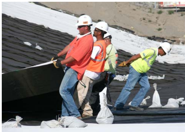
Liner installation at super cell 9
