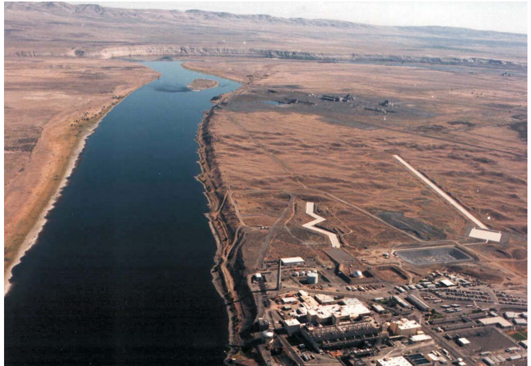
N Area included a total of 140 waste sites. They include sites of unplanned releases of contaminated material, as well as sites containing contaminated reactor piping, reactor hardware and other hazardous materials. In addition, reactor cooling water was disposed of in cement-covered trenches and cribs, pictured above.
