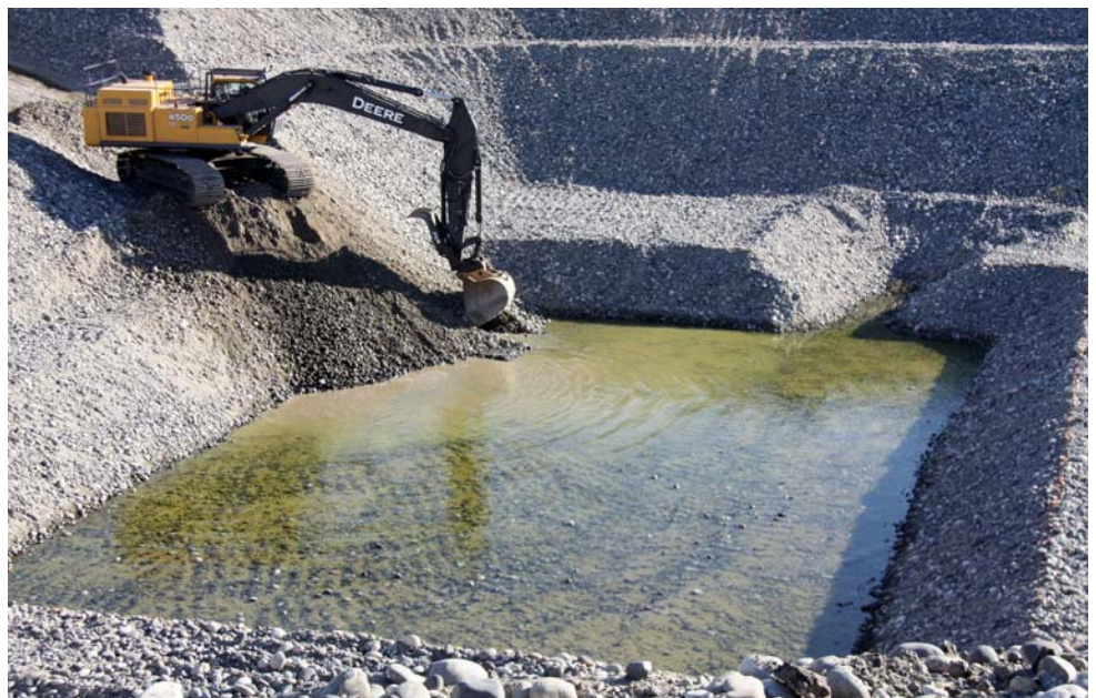
Washington Closure Hanford and subcontractor Ojeda Business Ventures excavate chromium-contaminated material from site 100-F-57 at F Area. The project team has excavated a plume approximately 42 feet to groundwater. The contamination is the result of leaks within the water treatment system of hexavalent chromium that was added to control corrosion in the piping for the reactor’s cooling system.
