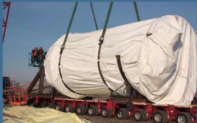
A special trailer for heavy loads was used to haul the CRCTA tank to the Environmental Restoration Disposal Facility. It took the crew several hours to slowly drive the Goldhofer trailer with its wrapped package to ERDF
