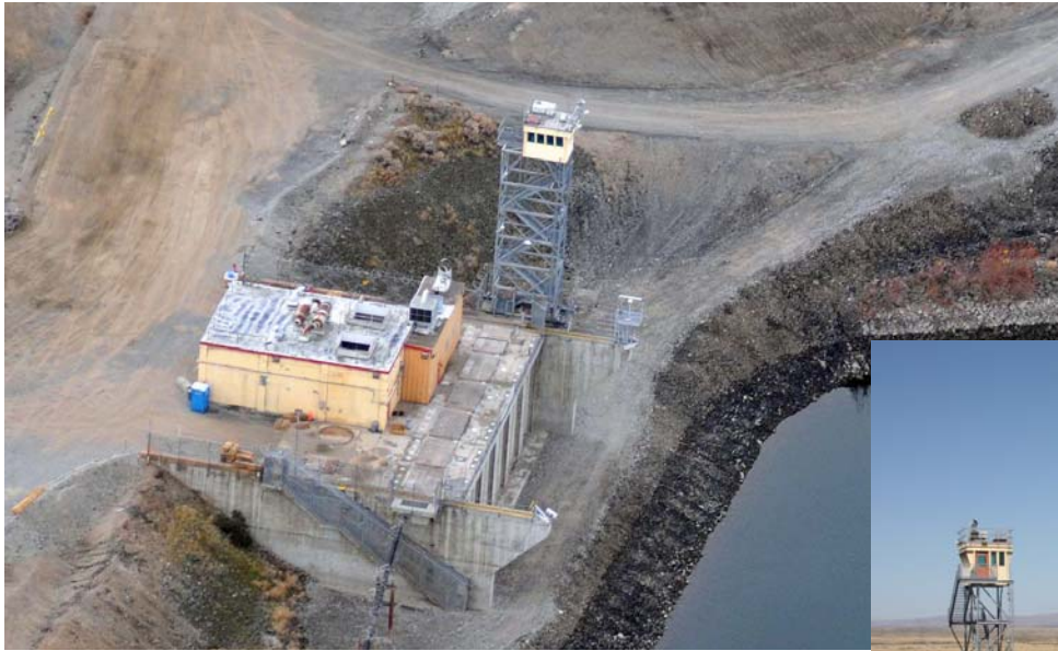
An earthen barrier was installed so demolition of river structures and the guard tower can be done safely.
