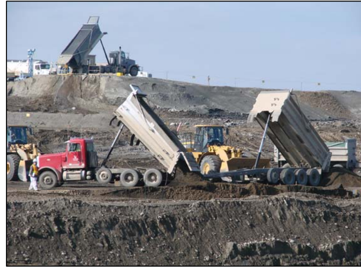
Truck-and-Pup and Super Dump ERDF Disposal Operations
