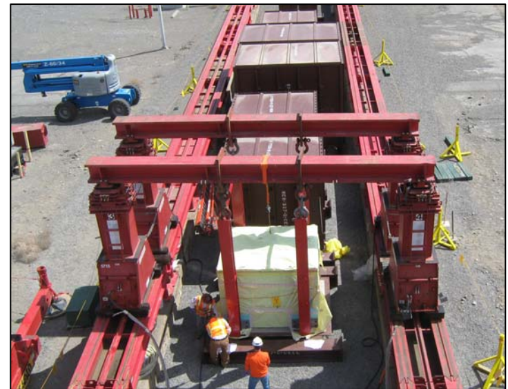
327 Facility Hot Cell Removal
