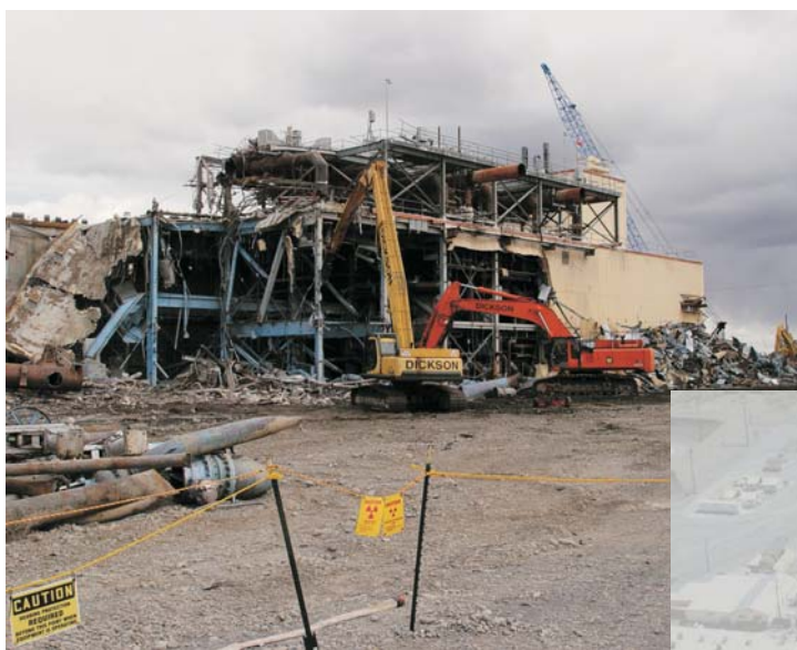
Demolition of the Heat Exchanger Building, 2009
