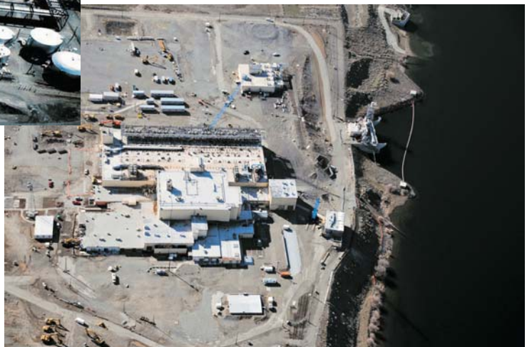
N Reactor, 2009. More than half of the 108 structures have been demolished.
