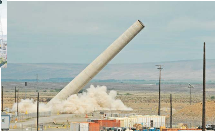
The main ventilation stack for N Reactor was demolished with explosives in June, 2008.
