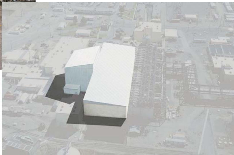
Conceptual drawing of cocooned N Reactor – complete by September 2012. When complete, 108 structures will be demolished and more than 150,000 tons of contaminated material will be transported away from the river.
