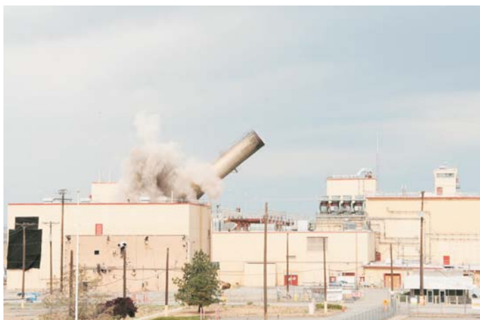
The N-Reactor powerhouse was demolished in June, 2008
