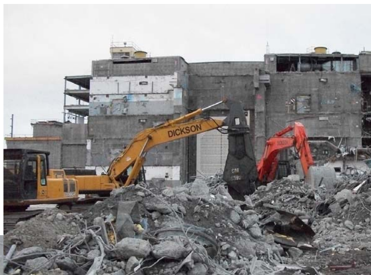
Demolition is underway on the north face of N Reactor, April 2010
