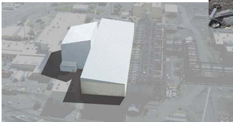
Conceptual drawing of cocooned N Reactor – complete by September 2012.
