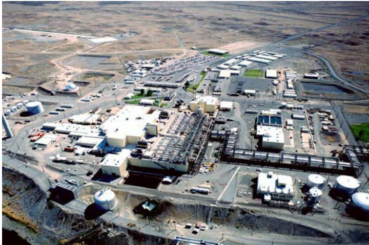
Operations ceased in 1987 and deactivation began in 1998. The N Reactor complex included 109 structures; 71 have been demolished
