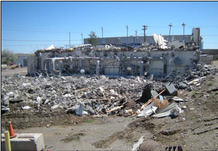
Demolition of 315 Complex
