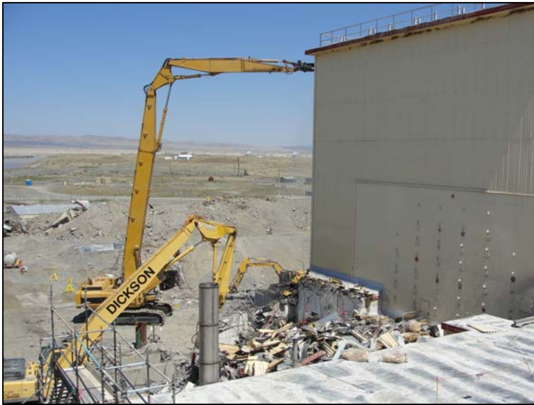
N-Reactor Demolition (west side)
