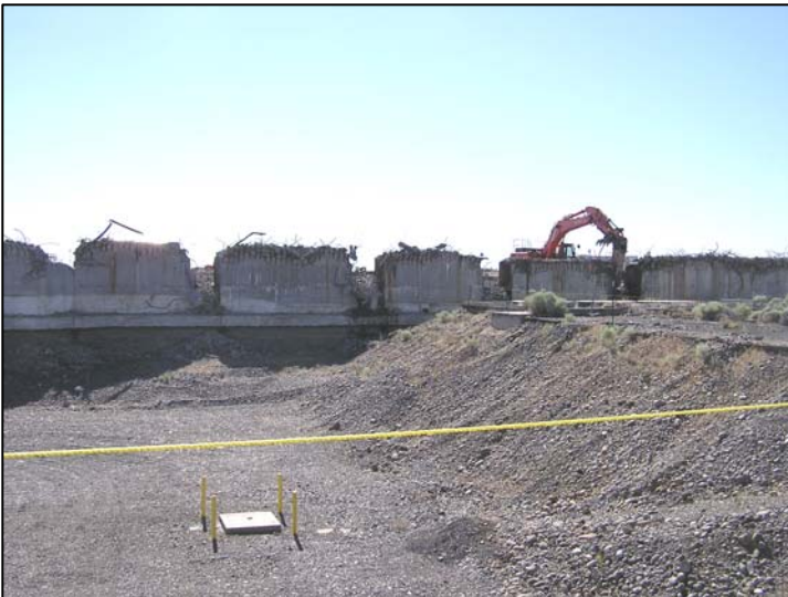
100-C-7 Concrete Wall Demolition
