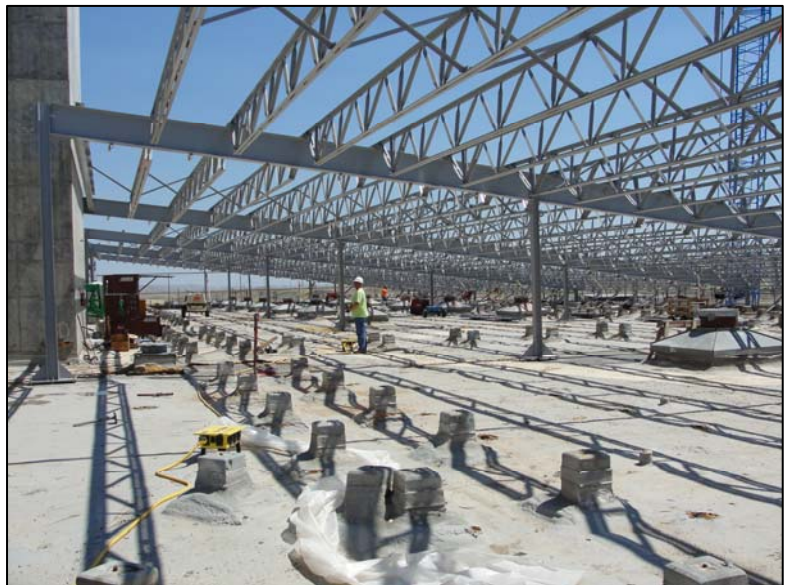
109N Safe Storage Enclosure Erection
