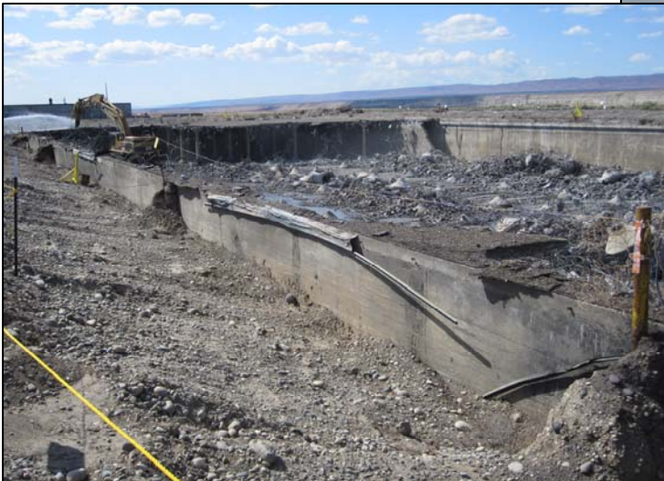
183H Clearwell Demolition
