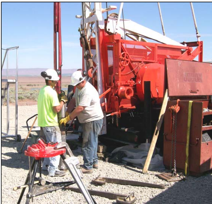
Recovering Vadose Zone Sample During RI/FS Well Drilling at 100-K Area
