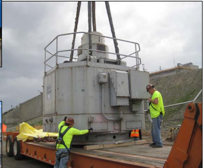
181N River Pump Motor Removal
