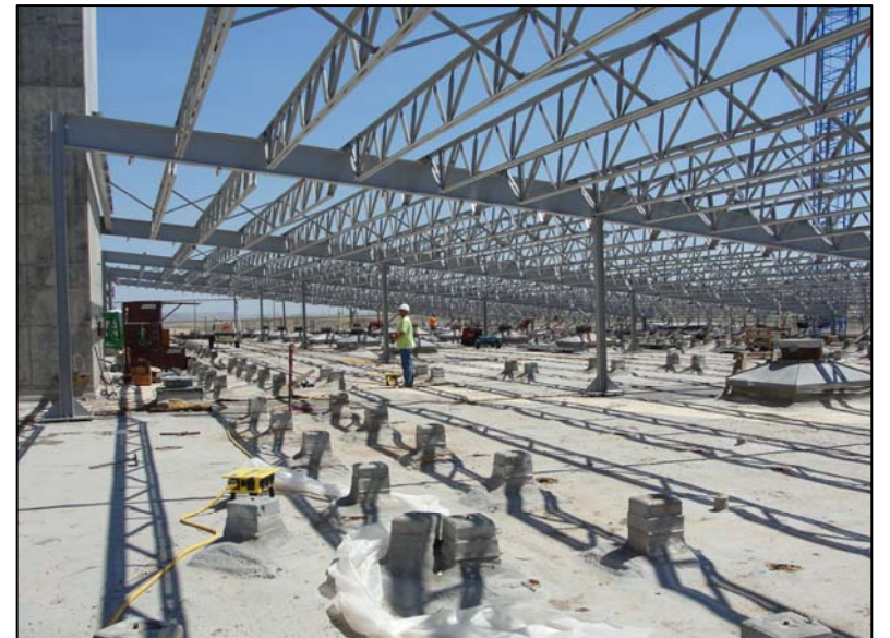
109N Safe Storage Enclosure Erection
