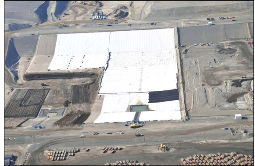
Super Cells 9/10 Liner Installation
