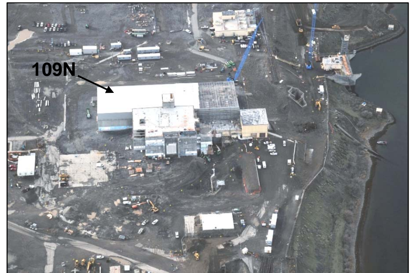
Roof Installation Nearing Completion on 109N ISS
