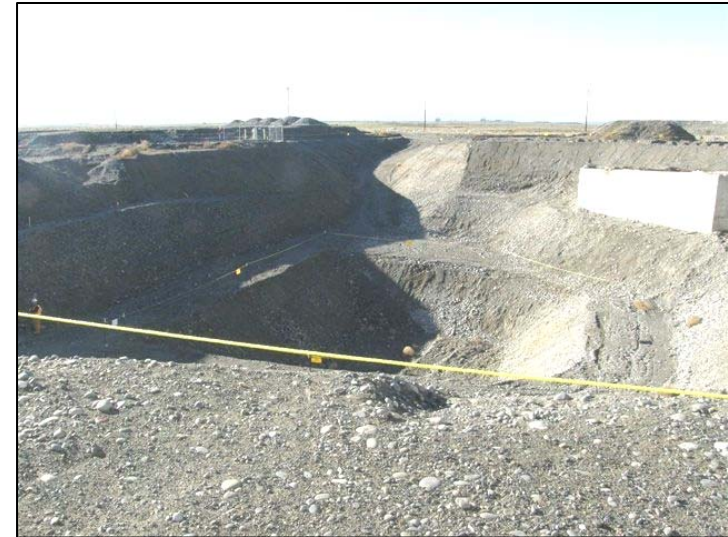
Completed 132-H-3 Excavation
