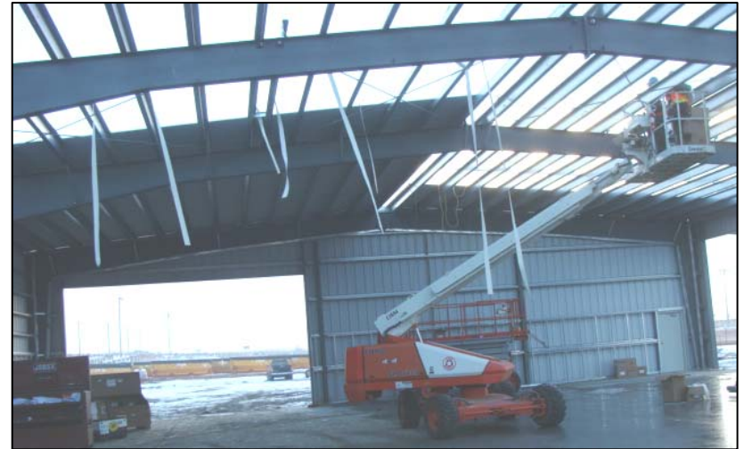
Installing Container Maintenance Facility Roof
