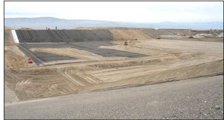
Super Cells 9/10 Construction Nearing Completion
