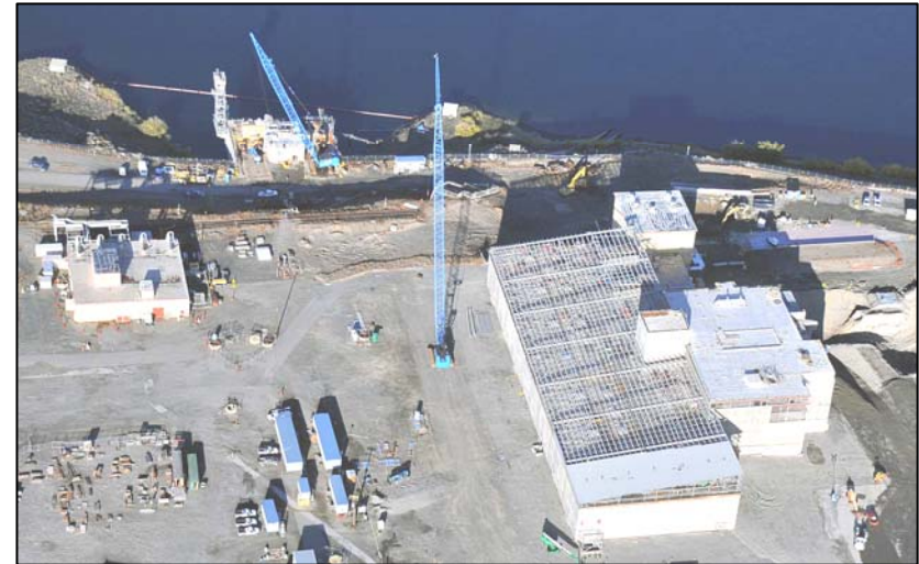
100-N Area -- 105N/109N Interim Safe Storage
