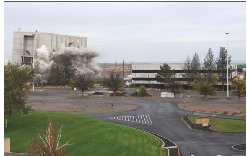
Explosive Demolition of 337/337B Buildings
