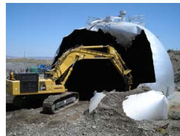
"Golf ball" waste facility demolition June 2009
