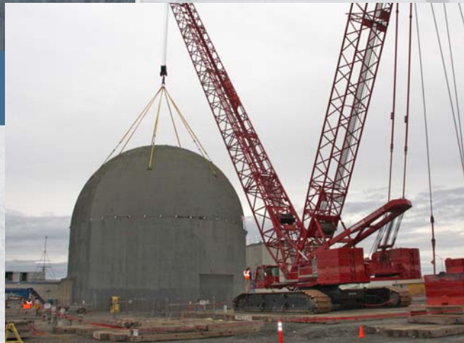
Workers monitor the 71-ton dome as it releases from 42 clips installed during the cutting process.
