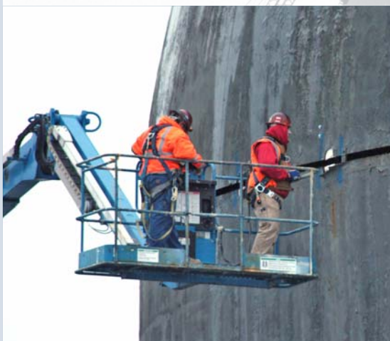
Workers monitor the 71-ton dome as it releases from 42 clips installed during the cutting process.
