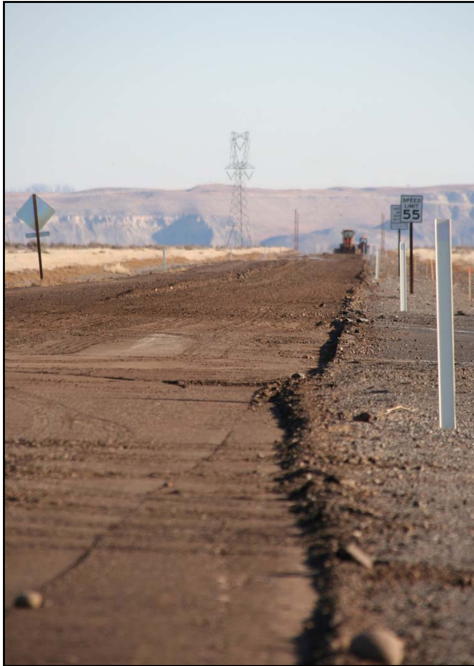
A 900-foot section of Route 1 is being prepared for paving.
