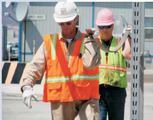
Mechanics Merrick Veit (left) and Mike Stoltz carry material used to help maintain Washington Closure's fleet of 600 containers, including 100 new containers placed in service this year.
