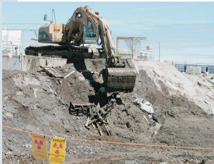
ERDF operations workers treated more than 32,500 tons of lead-contaminated soil from the 618-7 Burial Ground.
