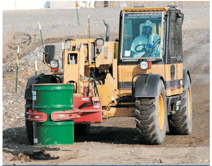
A worker at the 618-7 Burial Ground delivers a drum overpack to a secure enclosure for characterization. More than 800 potentially pyrophoric barrels were retrieved at the site.
