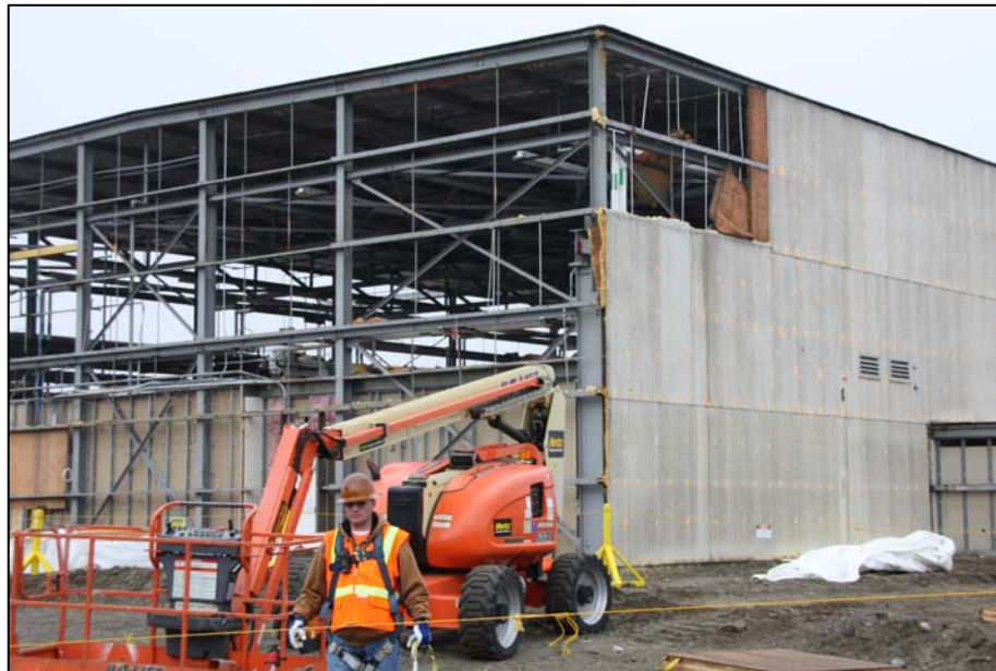
338 Maintenance Building Demolition
