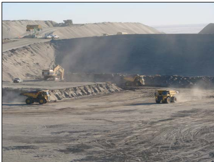
Excavation of ERDF Super Cell 9
