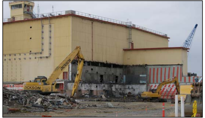
105N Control Room Demolition
