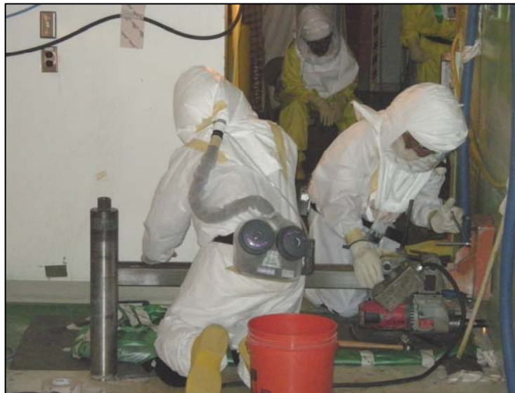
Core Drilling the 327 Building SERF Cell
