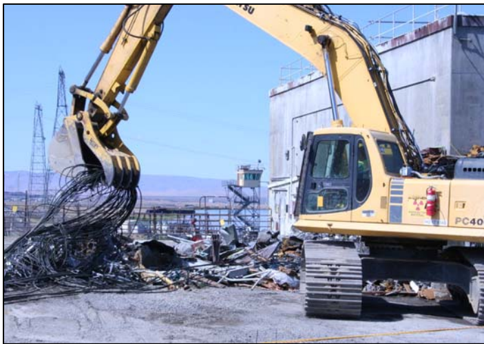
Demolition of 107N Building
