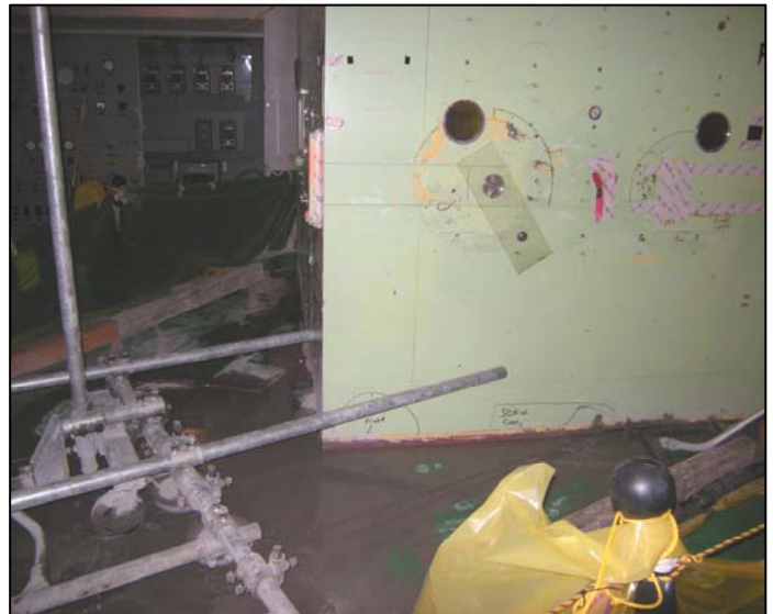
327 F Hot Cell Wire Saw Cutting (85% cut)
