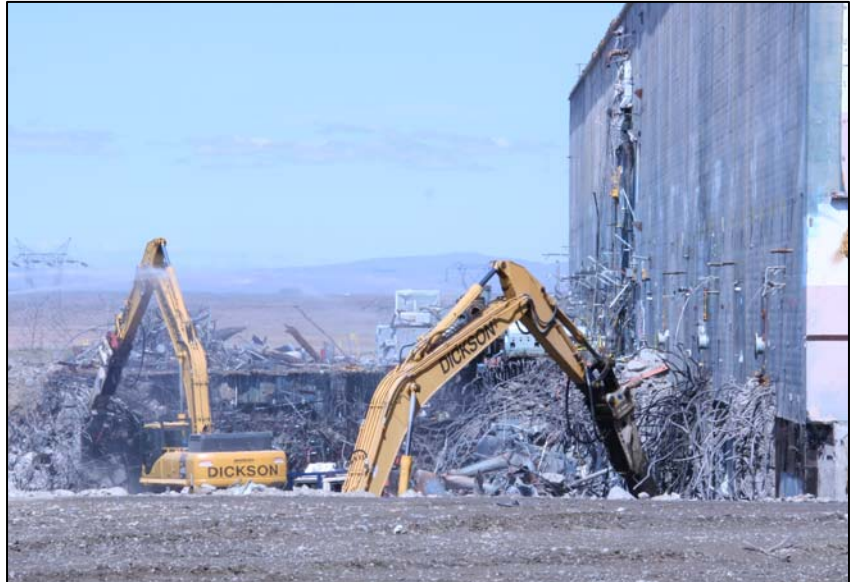
109N Below-Grade Demolition
