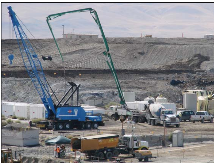
Void Fill Flood Grouting Operations at ERDF
