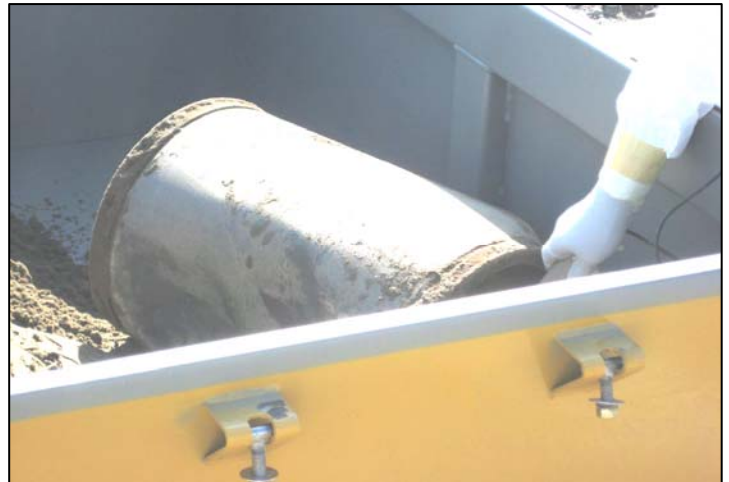
Anomaly Packaging of Drum Found Under 306 Building Slab
