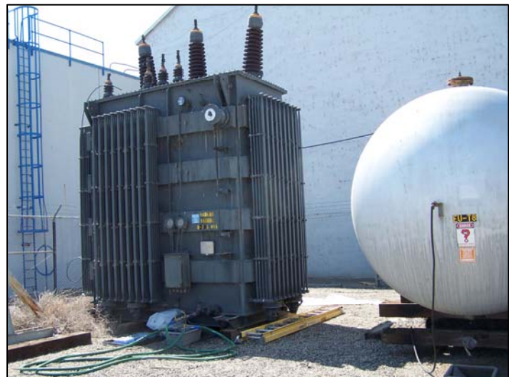
115kV Transformer - Drained ~4,700 Gallons of Oil Prior to 305 Building Demolition
