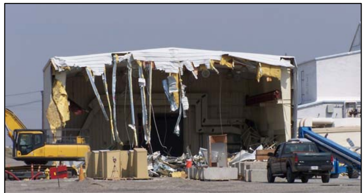
Demolition of 305B Hazardous Waste Storage Facility
