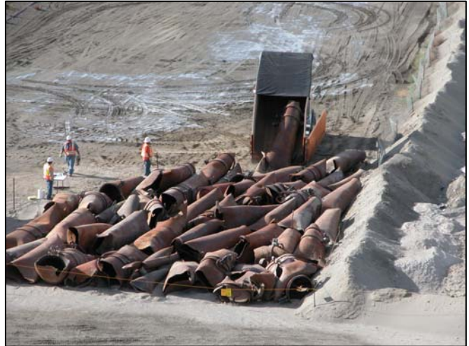
Placing 1802N Piping on the 0-Foot Level in ERDF Cell 5
