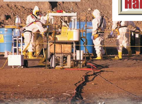
Reactor Interim Safe Storage
