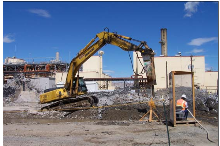
Hammering Foundation of 183N Water Filter Plant
