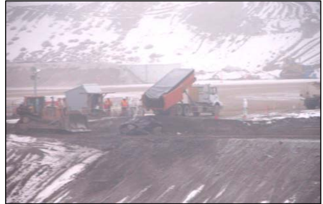
Dumping 300 Area Beryllium Waste in Cell 6 (during freezing fog conditions)
