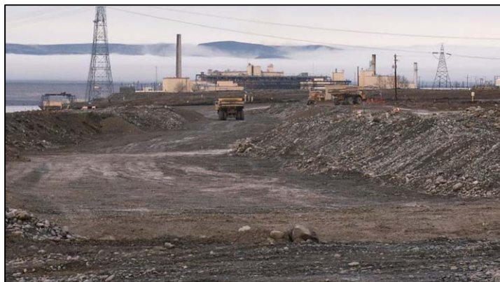
Backfill Activities at 116-K-2 Mile Long Trench
