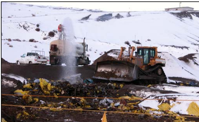
Compacting Beryllium Waste from 314 Building on Cell 5 Floor (water truck providing dust suppression)
