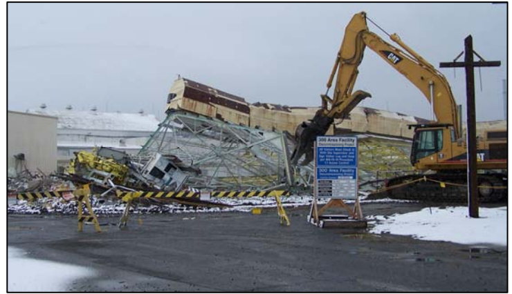
Cutting Up 314 Building Debris for ERDF Disposal
