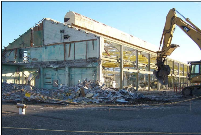
Demolition of 314 Building
