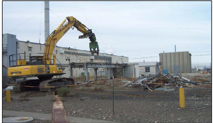
Demolition of 334TF Facility
