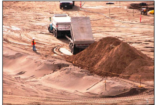
Dumping Waste Soil from Horseshoe Landfill in Cell 5
