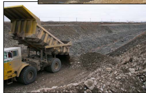
Backfill of 116-K-2 Mile Long Trench (east end)
