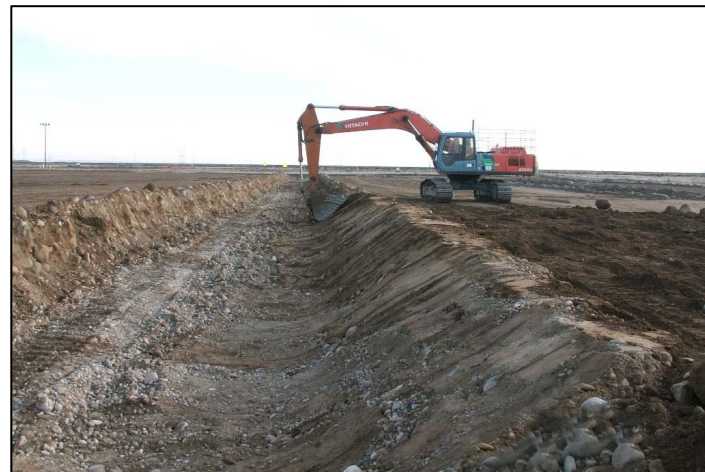
Constructing Sorting Trenches for 118-K-1 Burial Ground
