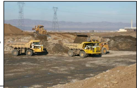
Loading Soil at Borrow Pit for 100-K Area Backfill Activities
