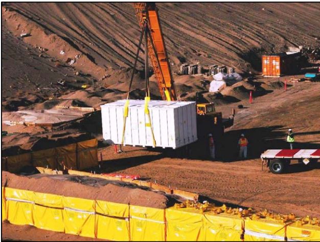
Offloading IP-II Container from K-Basins Containing Fuel Canister Storage Racks
