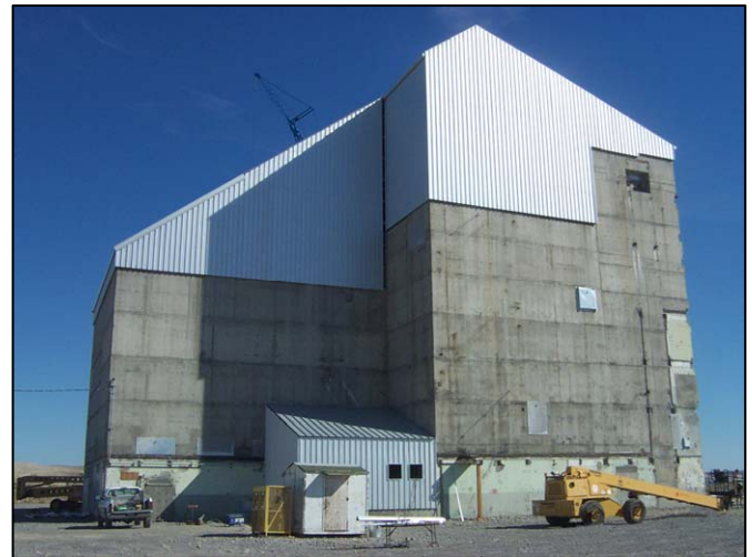
H Reactor - After ISS Completion
