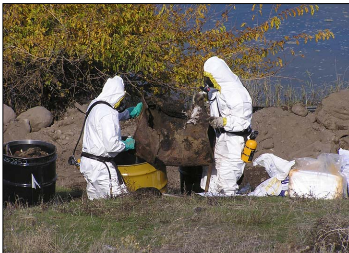
Transferring the Last of the Unknown Liquids from 128-B-3 into Overpack Barrel
