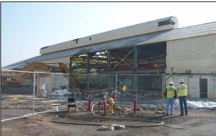
314B Demolition Loadout
