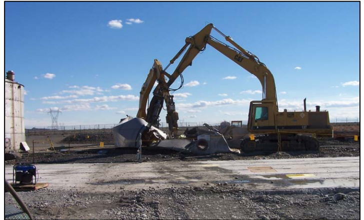
Demolition of 183-KW Alum Tank
