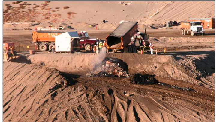
Waste Disposal at the 35-Foot Level of ERDF Cell 6
