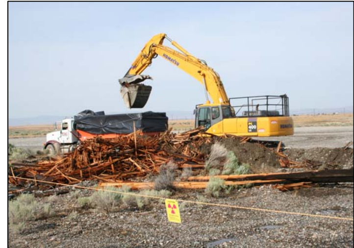
Loadout of Mud Dauber Contaminated Telephone Poles at 100-H
