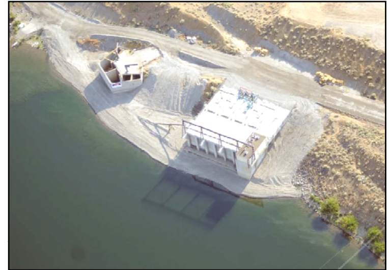
Bench Construction at 181NE and 1908NE
