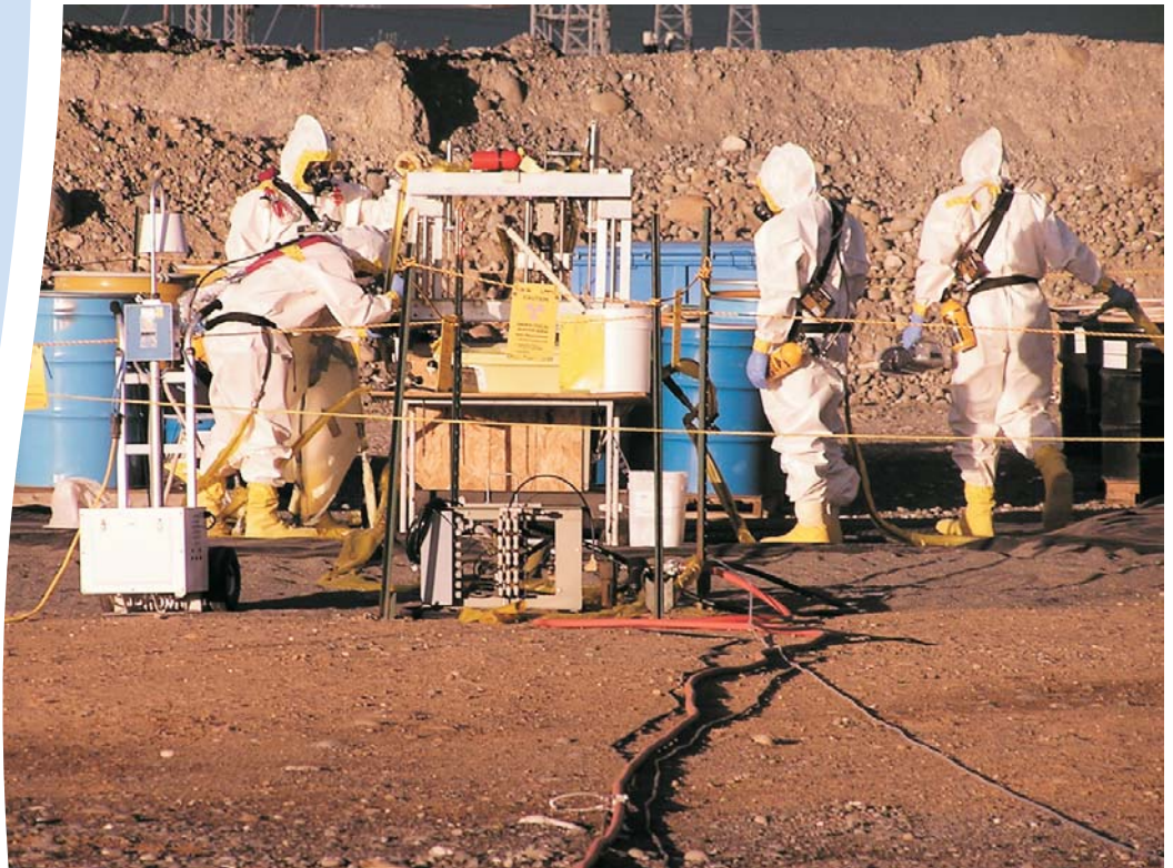
Field Remediation Project team members work in level-B protective gear as a precaution against contaminants, such as mercury, found in carbon steel tubes.
