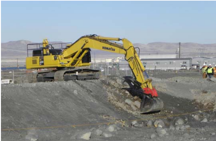
Anomalies are moved to a staging area for sampling
