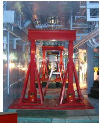
A gantry system was constructed for removal of the hot cells.
