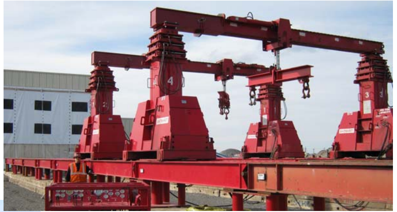
A gantry system was constructed for removal of the hot cells.
