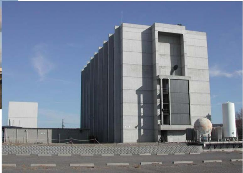
The 337B Building initially housed research and development activities associated with the Fast Flux Test Facility, including a reactor core mechanical mock-up, which was used to test selected FFTF components.
