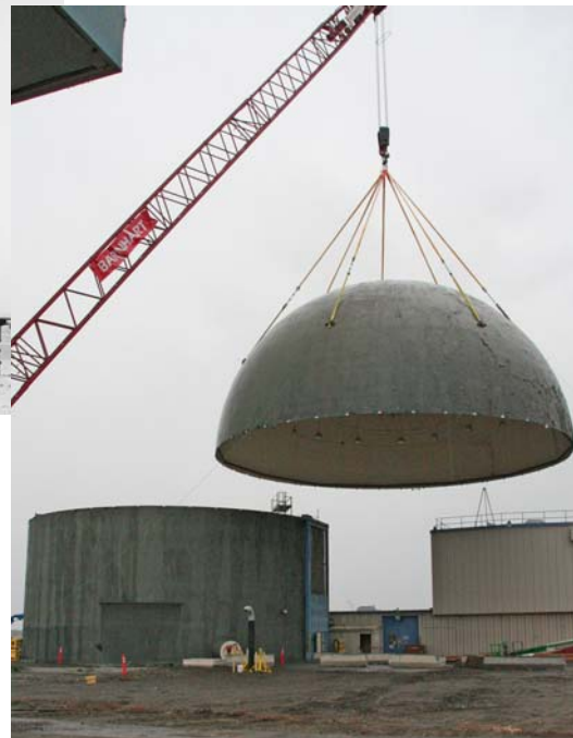
The 67-ton steel dome was removed January 15, 2011. Demolition of the above-grade walls will be completed this winter.
