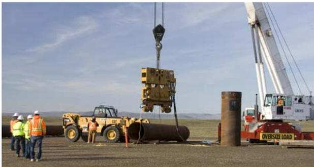
Project staff and stakeholders monitor the installation of a 48-inch over-casing to begin augering a drum style VPU.
