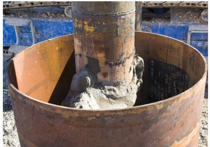
An auger was used to mix the simulated waste inside of the VPU, within a steel over-casing.
