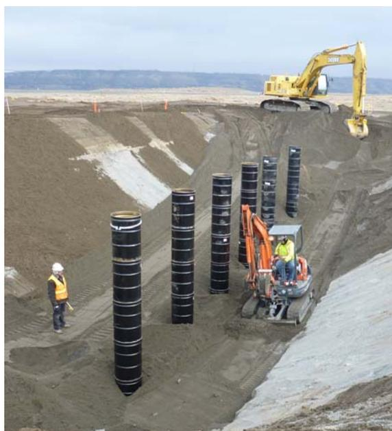
Simulated VPUs were constructed and buried in preparation for the method testing.
